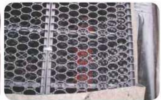
Typical tank installation format providing four clear access channels per every 400mm width
