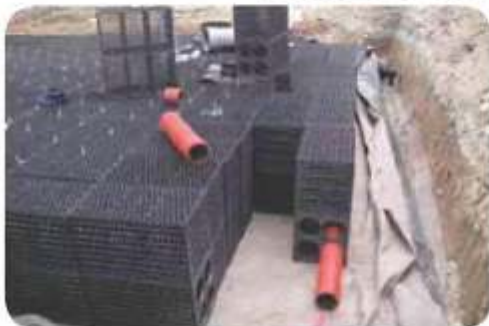
Typical tank installation format providing four clear access channels per every 400mm width
