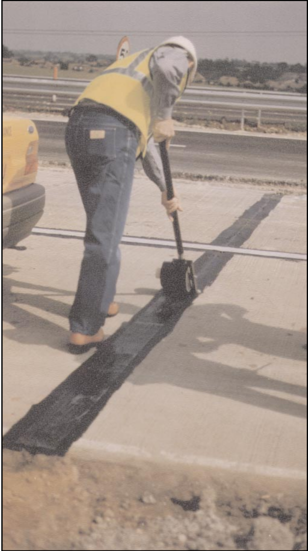
Applying Denso Paving Tape
