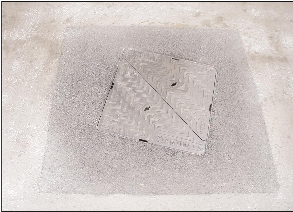
1. A new reinstatement ready for the application of Denso Overbanding Tape.
