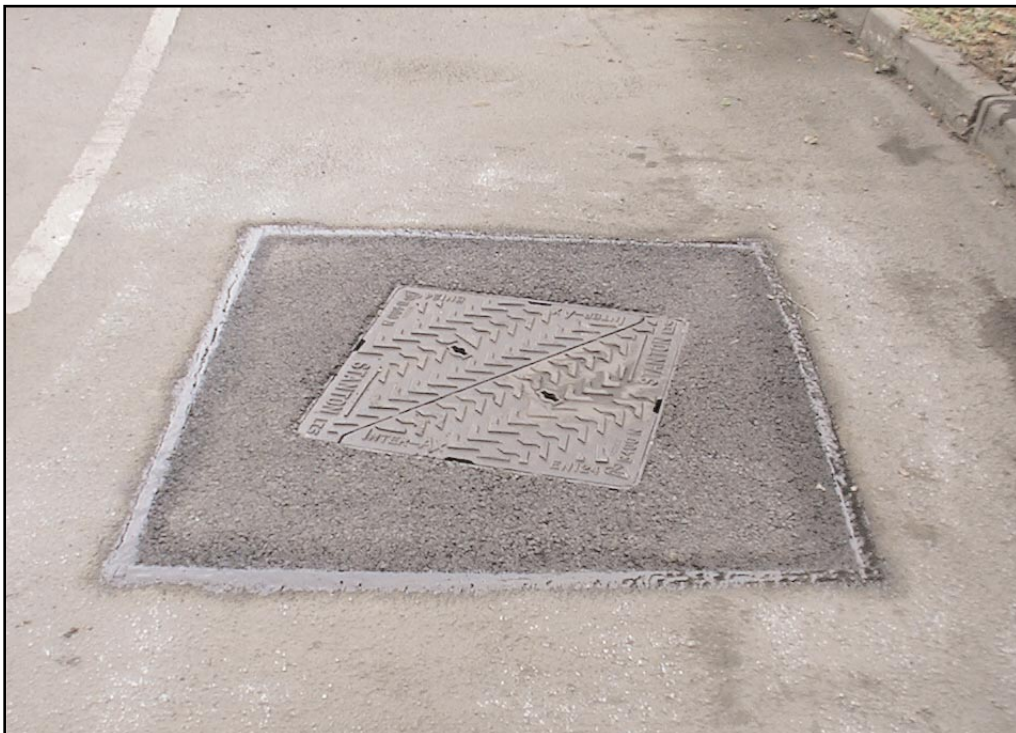
4. A finished reinstatement showing joint effectively sealed.
