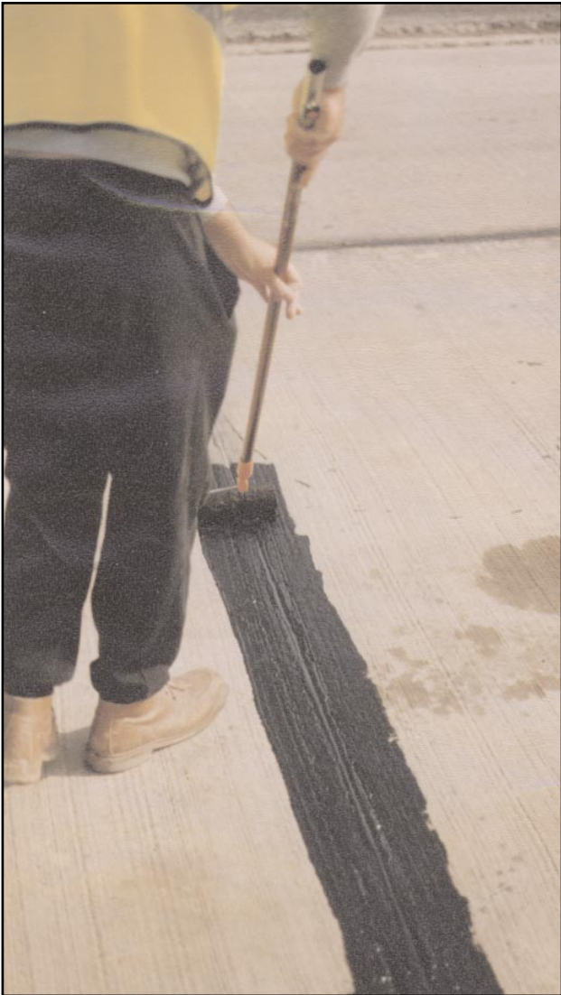
Applying Densoband Primer.
