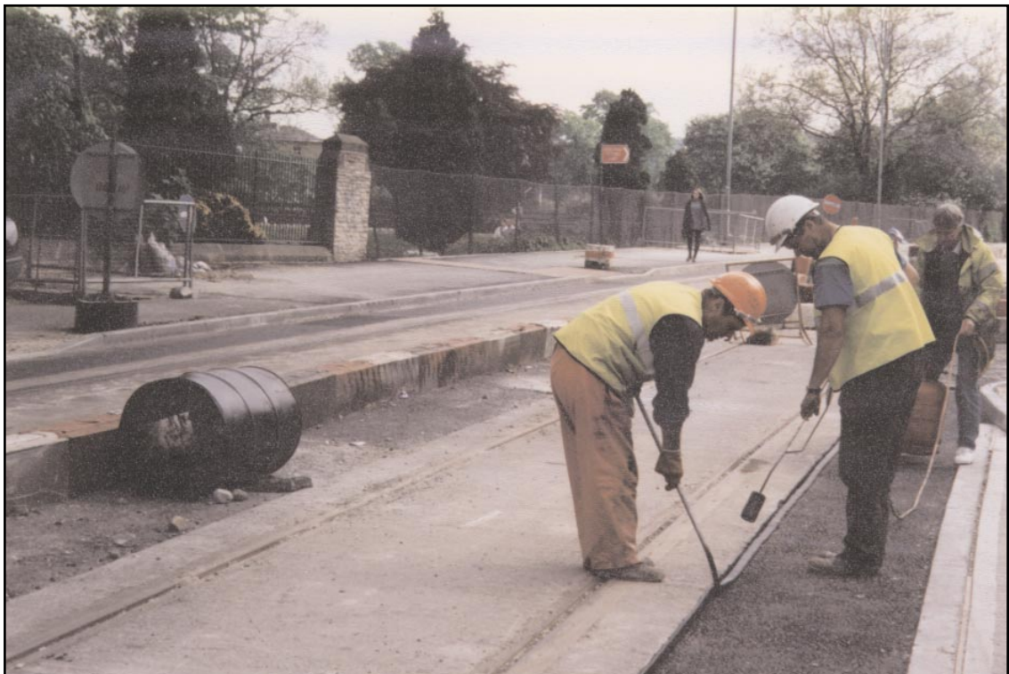
2. Hot application to vertical face of concrete tram rail bed.
