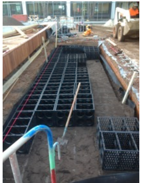
Installation of second layer of Ellipse modules. Note open internal panels
