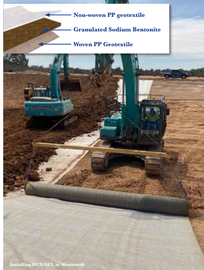
Installing DUX GCL at Wentworth
