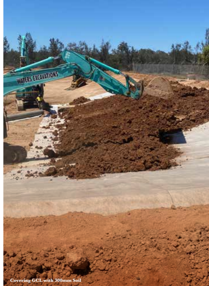
Covering GCL with 300mm Soil
