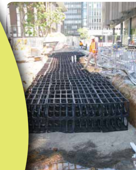
Terravault installed at Monash Transport Interchange, ready to be filled with soil
