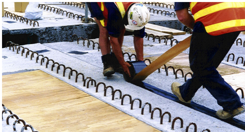
Placing 150mm Roadtape
