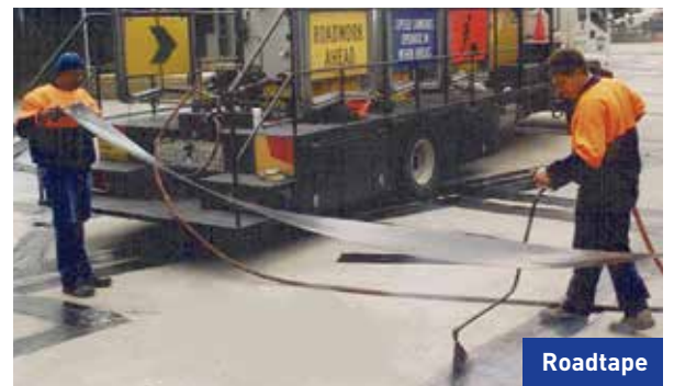
Placing 150mm Roadtape
