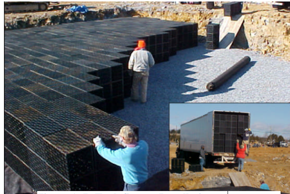
Figure 1: R-Tank System Installation
