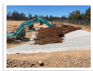
**DUX SPL40** GCL is a multi-component system made from a high-tensile PP woven base, internal
