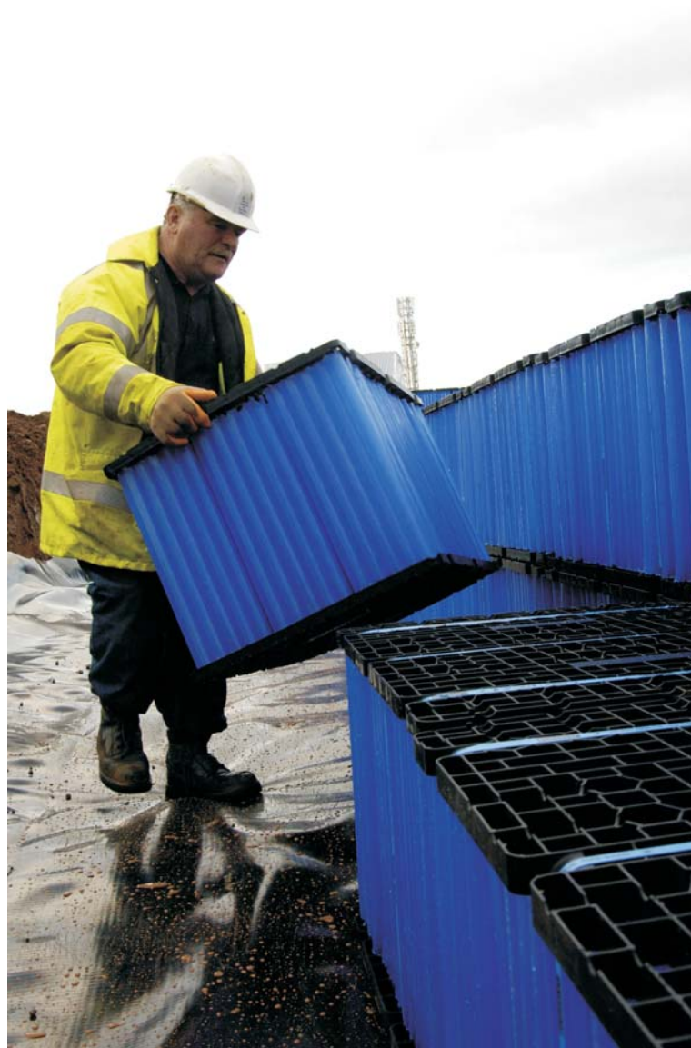
Modular geocellular units are lightweight and easy to handle
