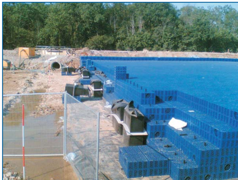
Figure 1.1 Large attenuation tank constructed from individual geocellular units
