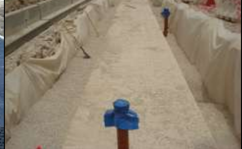
BACKFILLING
