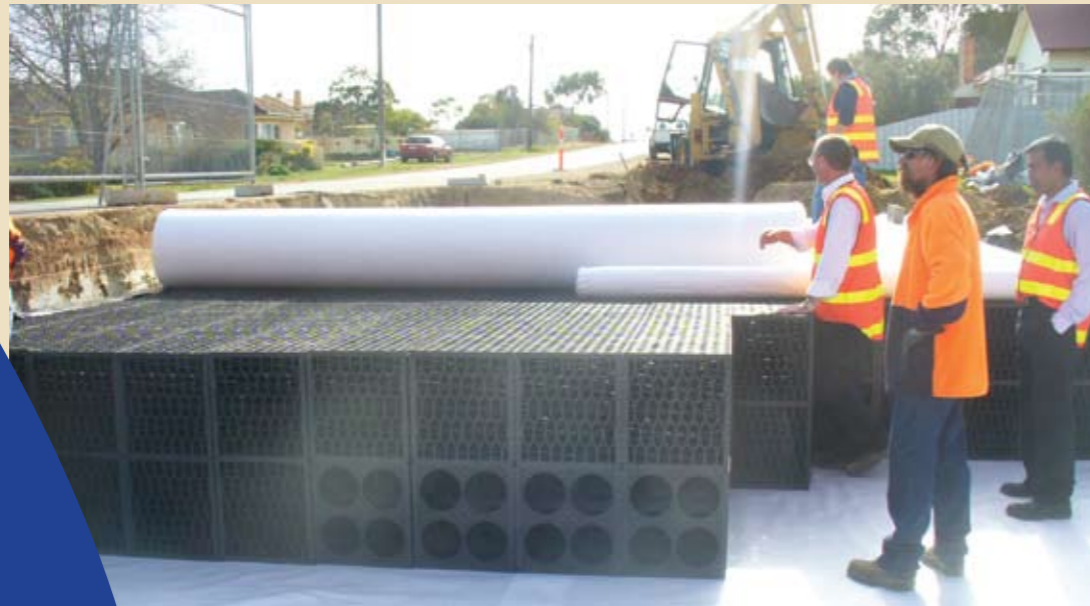
Installing Flushable Ellipse modules at Grant Street, Stawell
