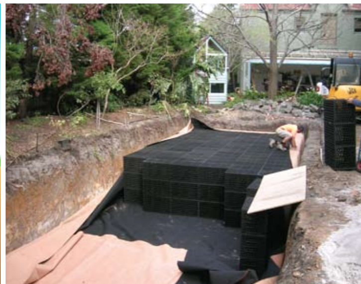
RainBox® underground water tank system; Absolutely Underground installing RainBox® 80kL tank at Toorak.
