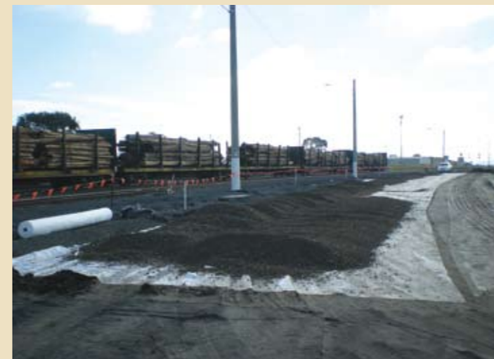
DUX® 56c installed under sub-ballast at Geelong railyard.
