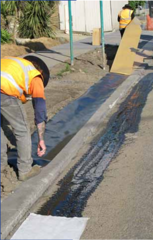
SIMPLE "PEEL AND STICK" ROADGRID INSTALLATION
