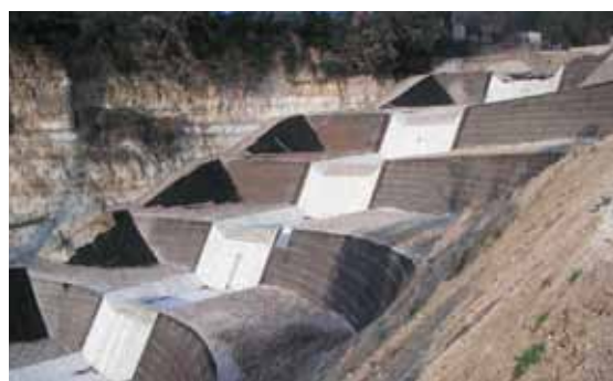
SPILLWAY CONSTRUCTED WITH FORTRAC-REINFORCED BENT STEEL MESH
