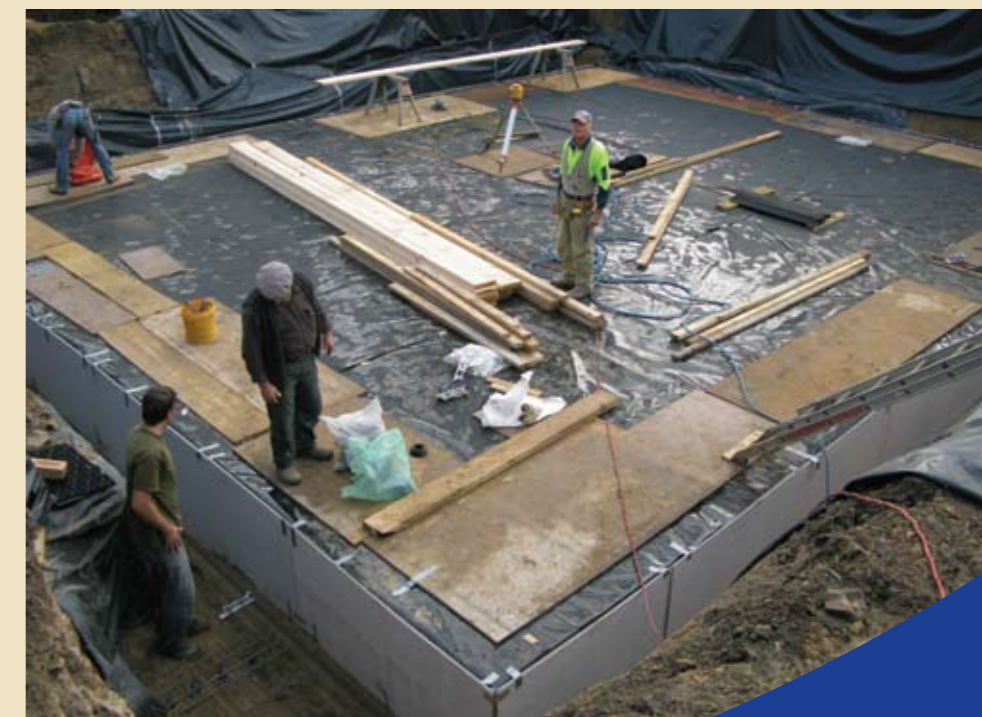
Preparing for the concrete pour around the Matrix® double modules.
