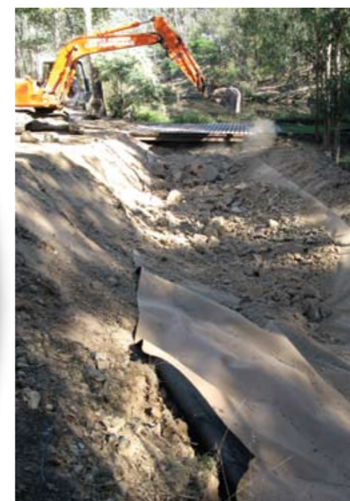
Placing CANAL3® in dam spillway
