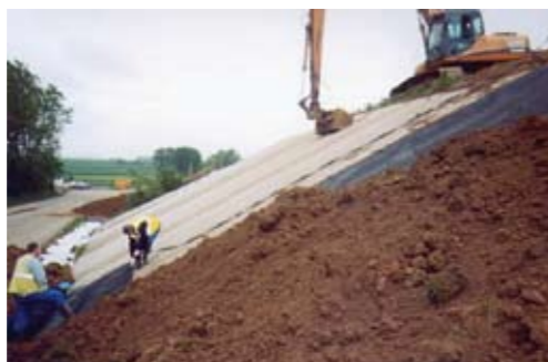
Installing Fortrac 3D® at Landfil de Curgies, France
