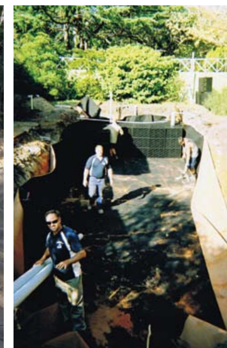
Installing CANAL3® with modular underground water storage
