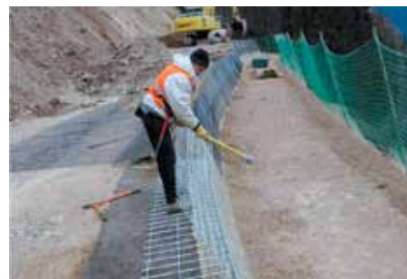
CONSTRUCTING STEEL MESH FACE WITH FORTRAC GEOGRID SOIL REINFORCEMENT
