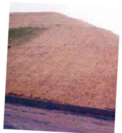
STEEP SLOPE TREATED WITH MAT
