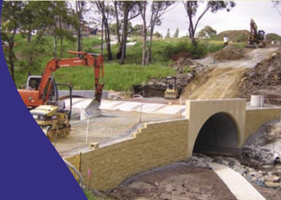
Tasman walls taking shape around concrete bridge arch
