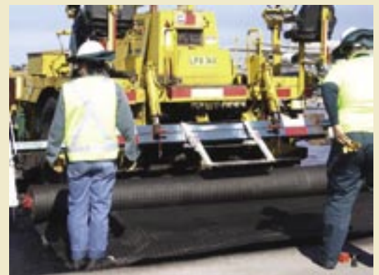
Laying Hatelit C at Sydney Airport
