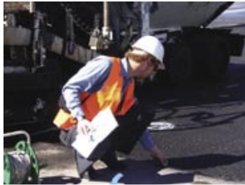
Matt inspecting Hatelit C installation at Sydney Airport
