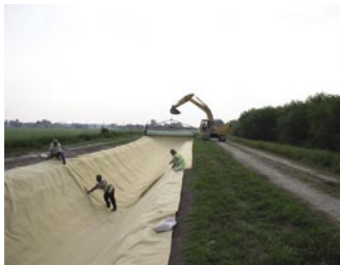
Installation of Canal 3
