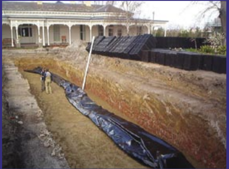
Ready to begin installing the 420 Matrix Quad modules
