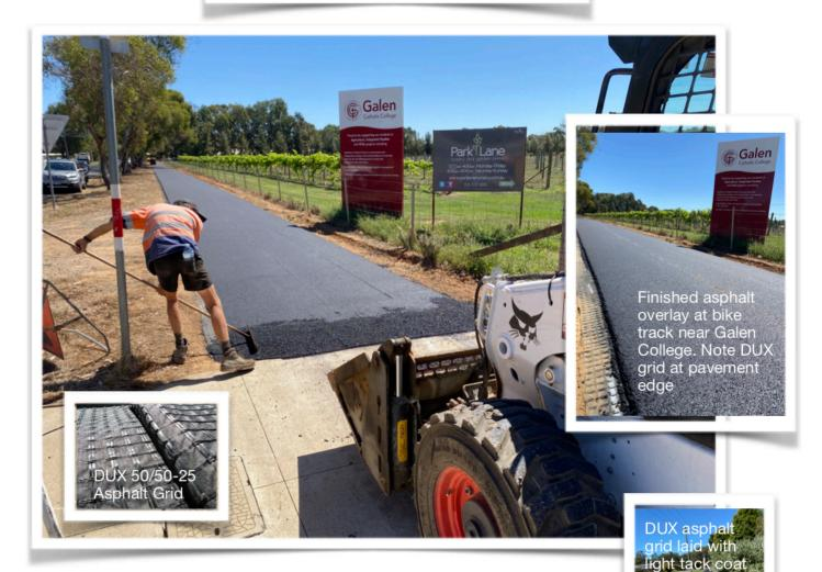
There is nothing like the crackling sound of freshly laid asphalt! Ensure your bike path achieves its' design life by including a layer of DUX asphalt grid in the overlay. DUX 50/50-25 is a specially designed polyester geogrid, combined with an ultralight PP non-woven that intercepts and deters reflective cracking. Recent bike path projects at Shepparton and Wangaratta show the word is spreading.
