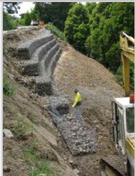
Geogrid-reinforced Gabion-faced wall
